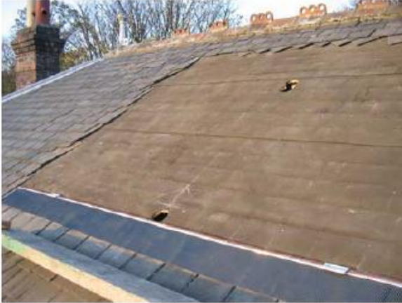
Slate roof without battens
