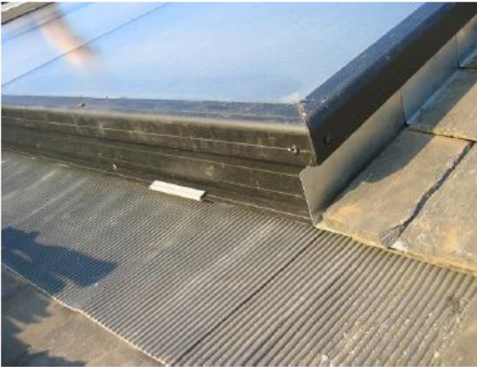
Place soakers and slates starting at the lead bib
