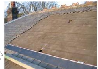
Slate roof without battens
